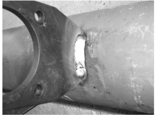
Figure 6. Final S-cam bracket weld
